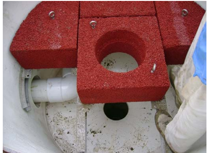
Installation of block segments inside portable unit.
