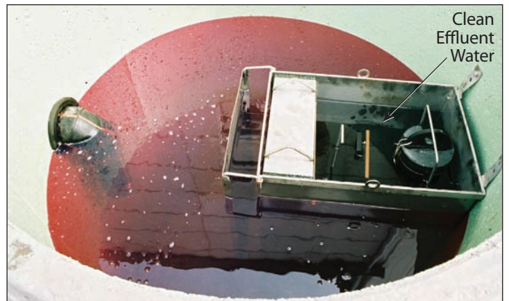
ecoLine™-b in operation with heavy oil loading on water surface
